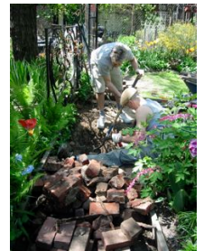
Volunteers Tom and Stephen successfully construct a dry well.
